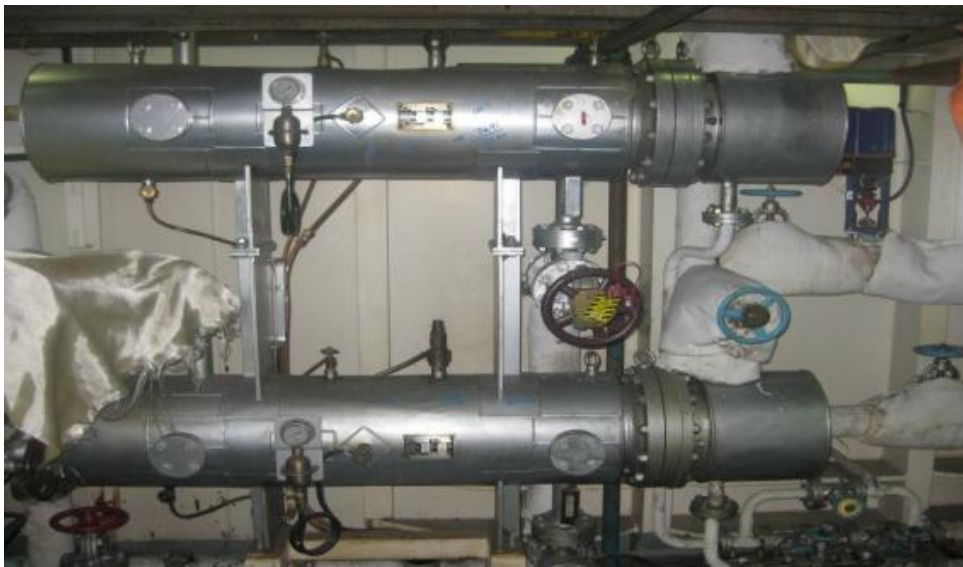
Figure 6.4: Typical fuel oil heaters
