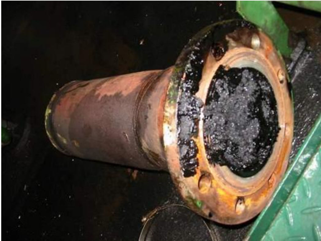
Figure 6.1: Clogged fuel pipes due to very poor-quality fuels
